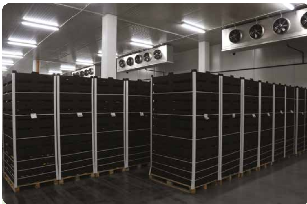
Figure 1 - Storage chambers set at 0-1^{\circ}\text{C} for apples and chilling-insensitive fruits.
